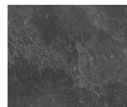
Black Concrete A B C
