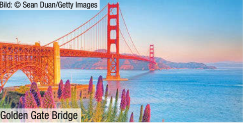
Golden Gate Bridge
